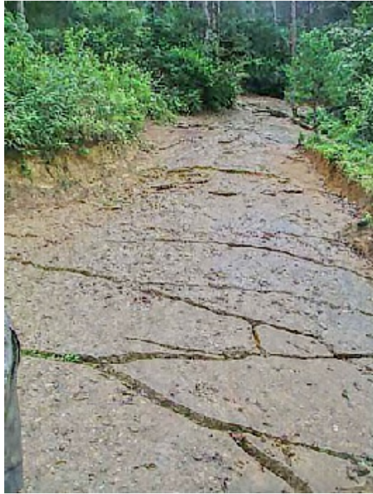
Image 4: Another section of concrete slab excavated on the north side of the pyramid. (P. LaViolette © 2014)
